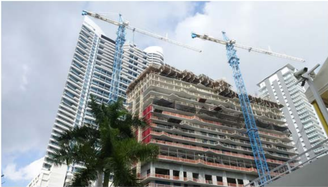
SLS Brickell under construction; The Related Group of Florida (Developer)
