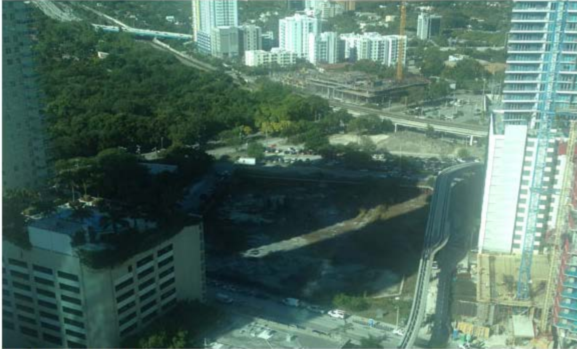
Former Capital at Brickell site
