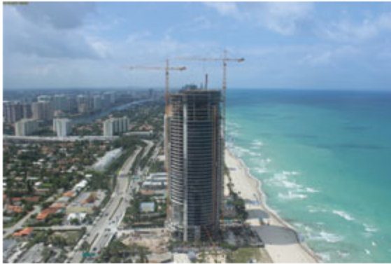
Porsche Design Tower under construction; Dezer Development (Developer)
