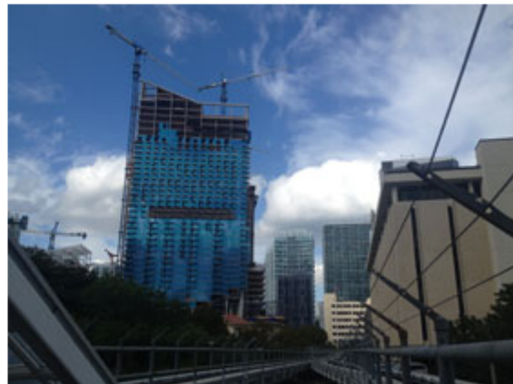
On-going construction of EAST, Miami within the Brickell City Centre Complex
